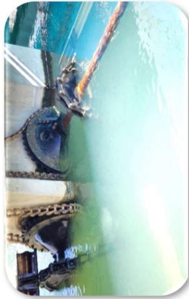
Project Description: This project will replace the existing chains and flights of the sludge collection and removal system for sedimentation basins at Plant “B”.
