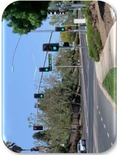
**Project Description:** This project will improve signal hardware including lenses, backplates with retroreflective borders, mounting, size, and number. This will also install pedestrian countdown signal heads and install an advance stop bar before cross walk.
