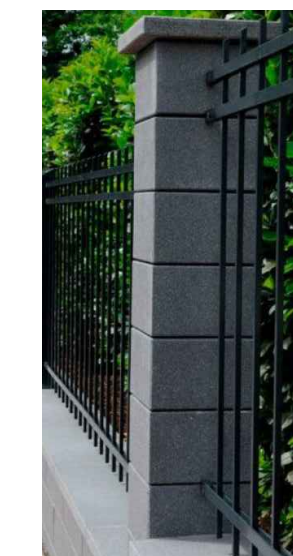
BLOCK PILASTER WITH PRECAST CAP AT MAIN ENTRY.
