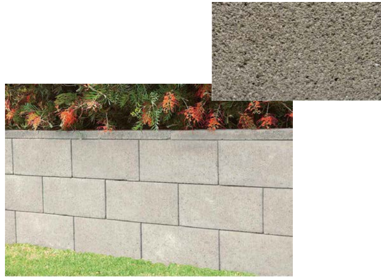
CMU BLOCK RETAINING WALL. COLOR TO BE EARTH-TONED/TAN. REFER TO CIVIL ENGINEER'S PLANS FOR HEIGHTS.
