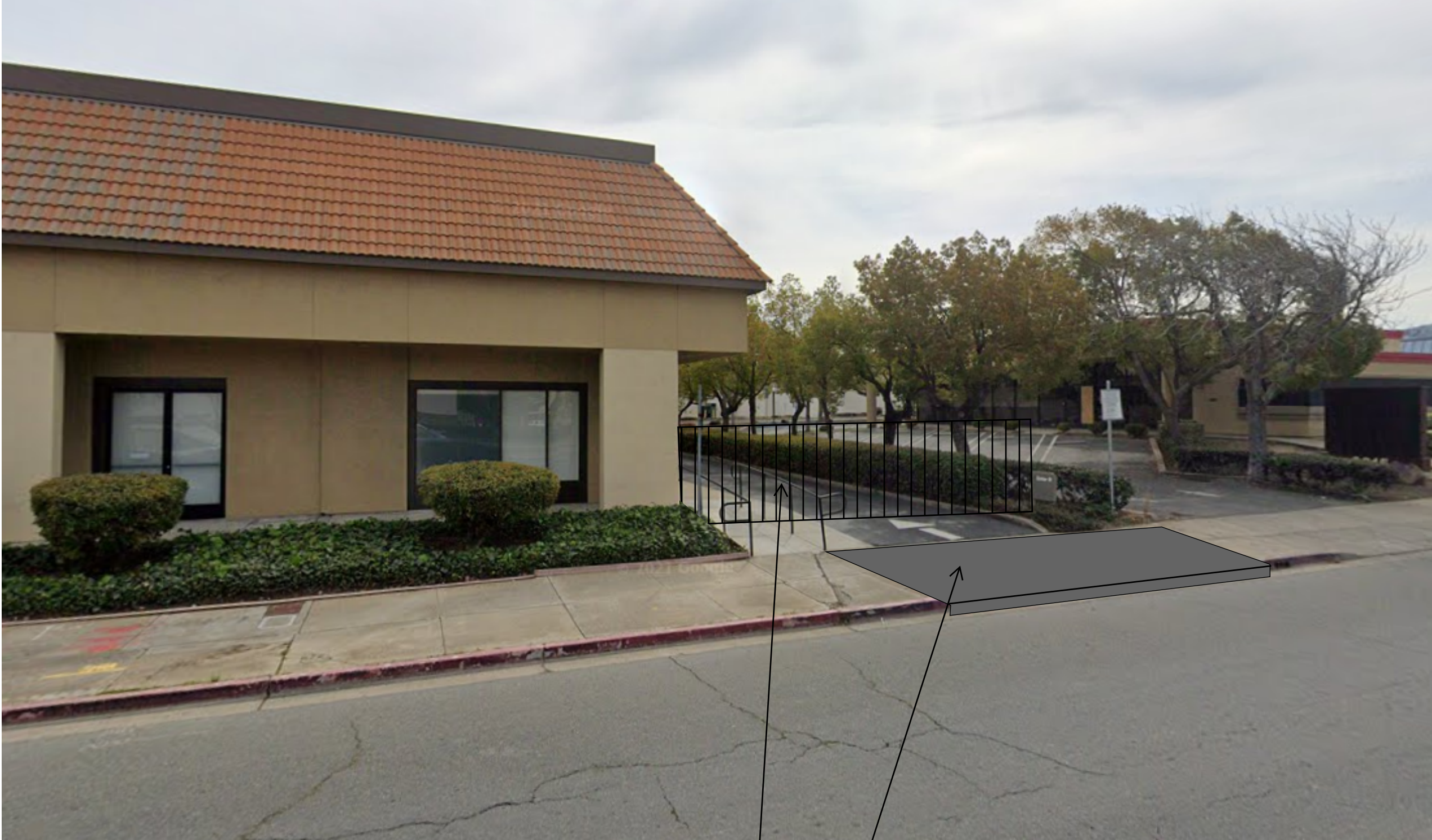
Somersville Rd Frontage
