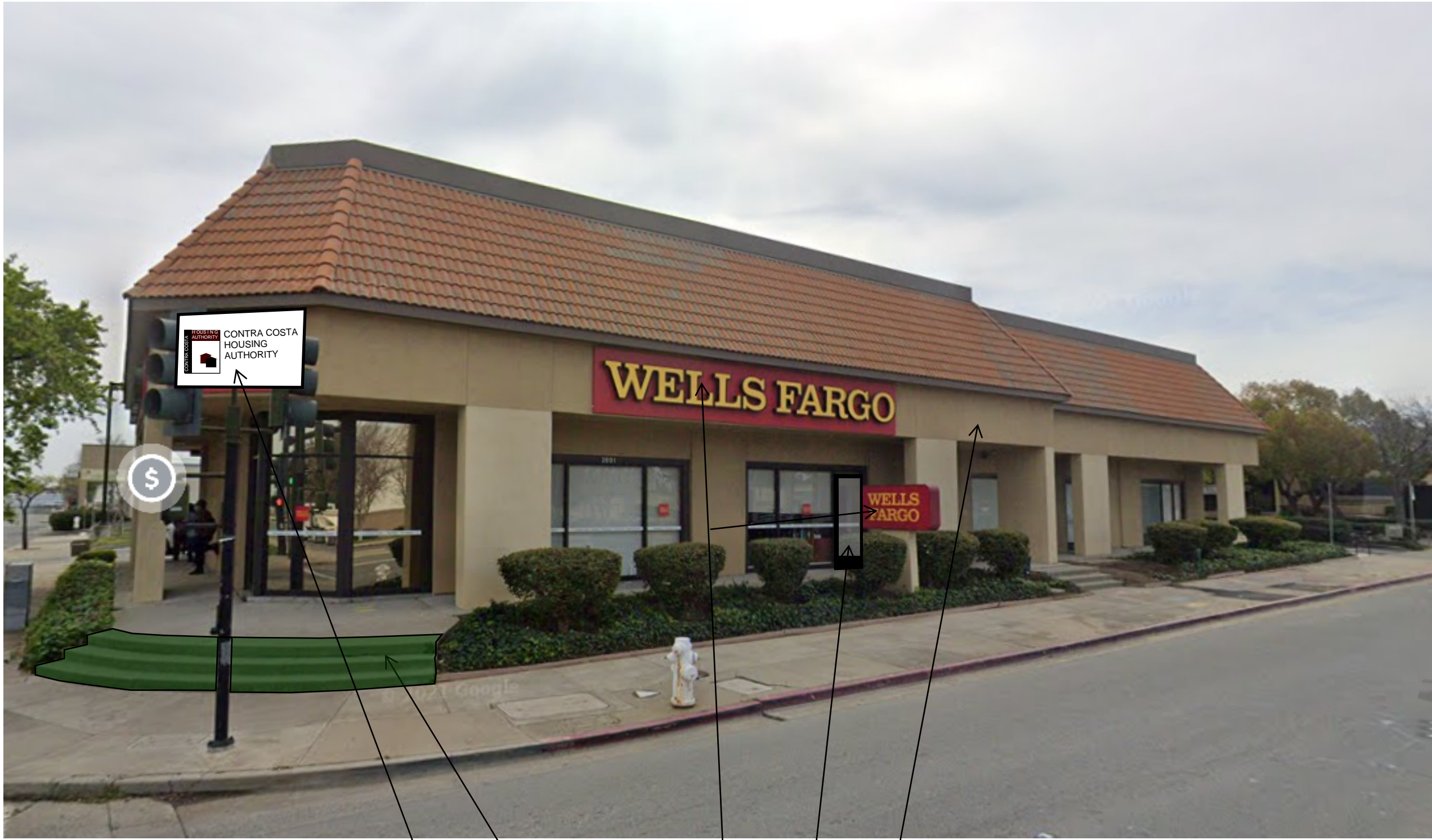
Somersville Rd Frontage
