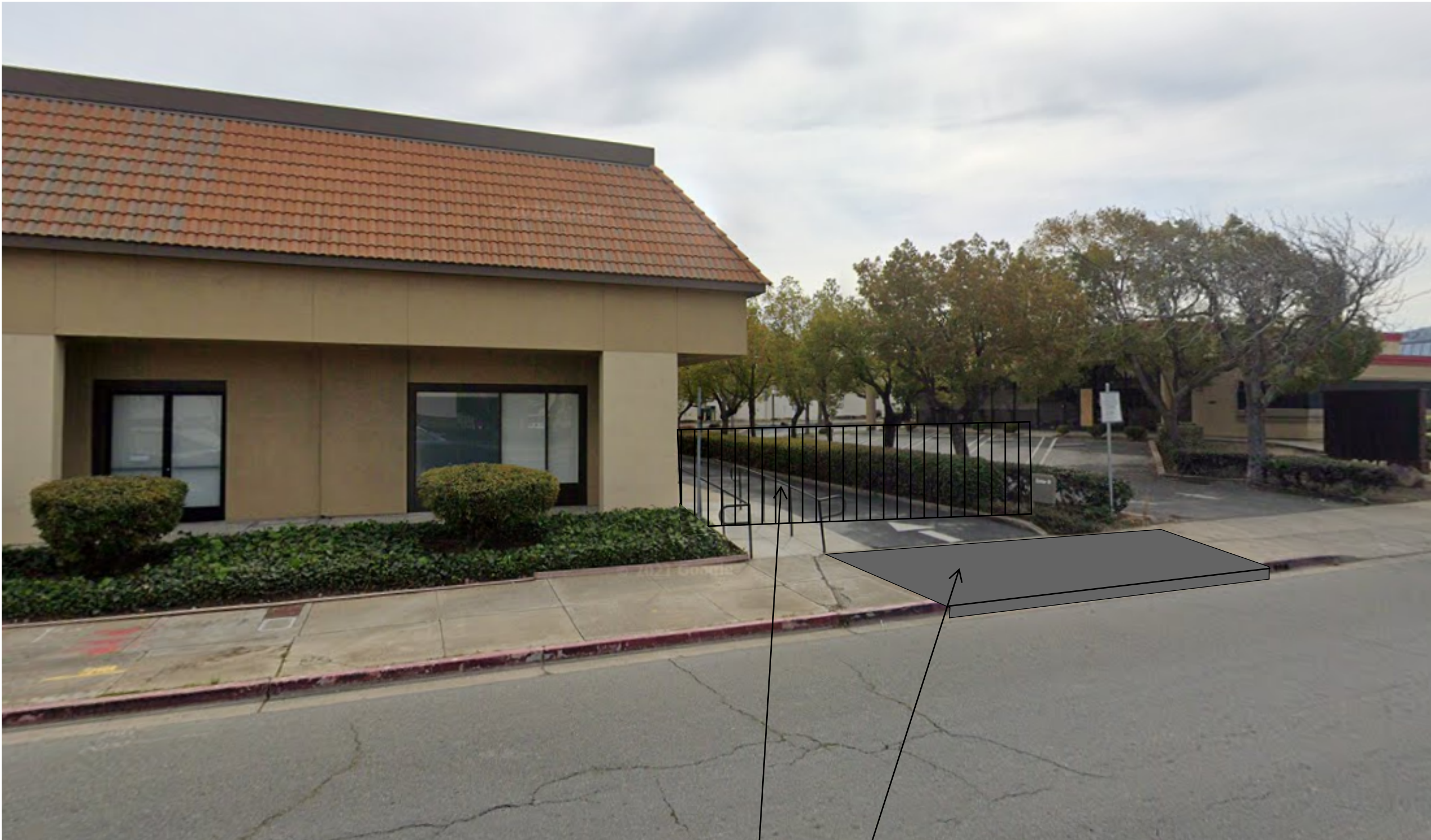
Somersville Rd Frontage
