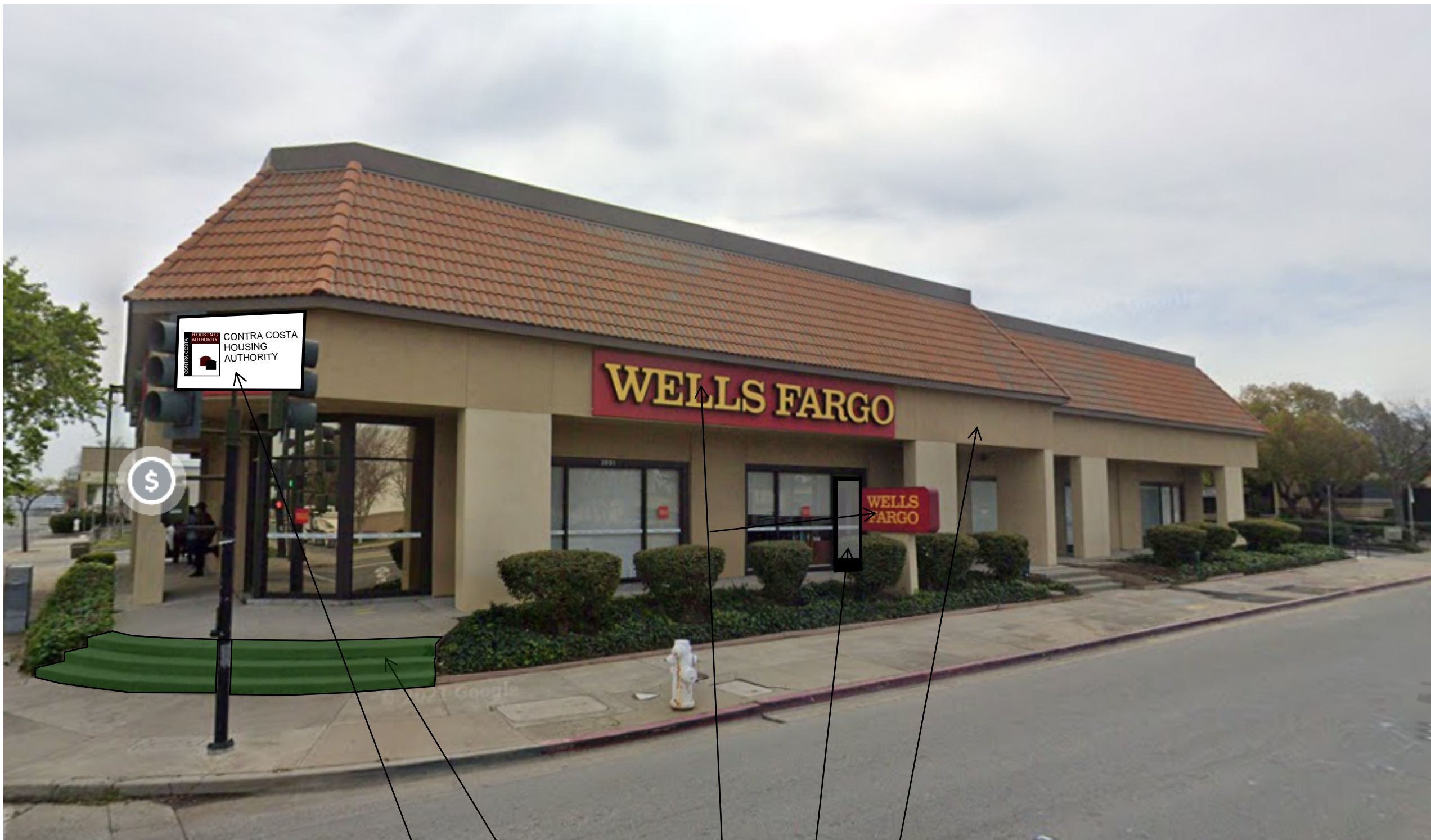
Somersville Rd Frontage
