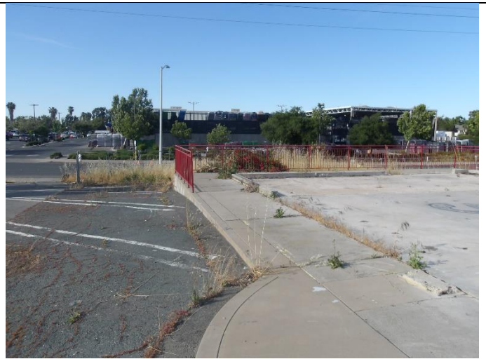
Leftover foundation slab with fence (will be demo)
