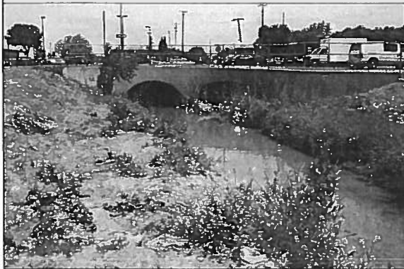
Figure 1. Canal, south of 10 th Street, view north.
